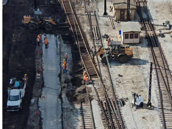
Converting Yard Track to Mainline
